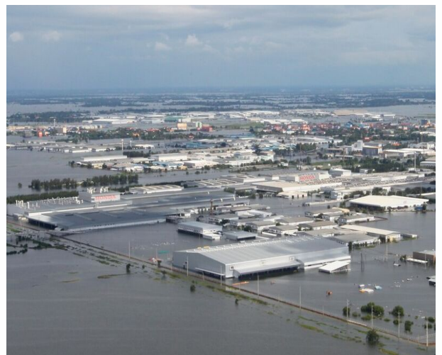
Floodwaters inundated Rojana Industrial Park in Ayutthaya Province, Thailand, in the 2011 floods. (Credit: Cpl. Robert J. Maurer via Wikimedia Commons)
