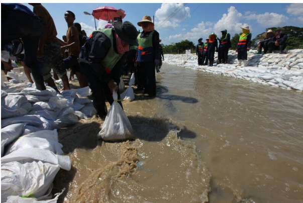
Volunteers and members of the Royal Thai Army, military police, fill and place sandbags to redirect flooding in the northern Sai Mai district in October 2011. (Credit: Cpl. Robert J. Maurer via Wikimedia Commons)
