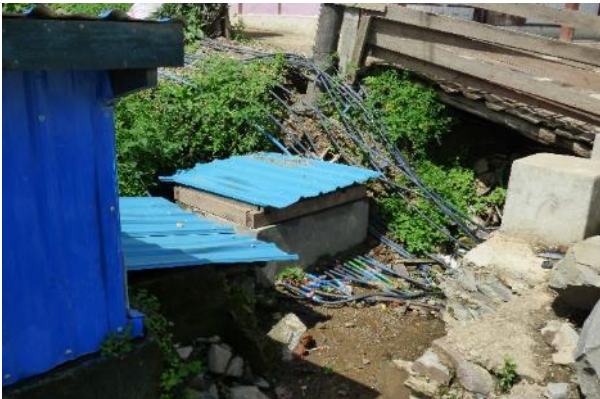
A spring source that distributes water to multiple houses in a block in the town (Credit: Carl Middleton)
