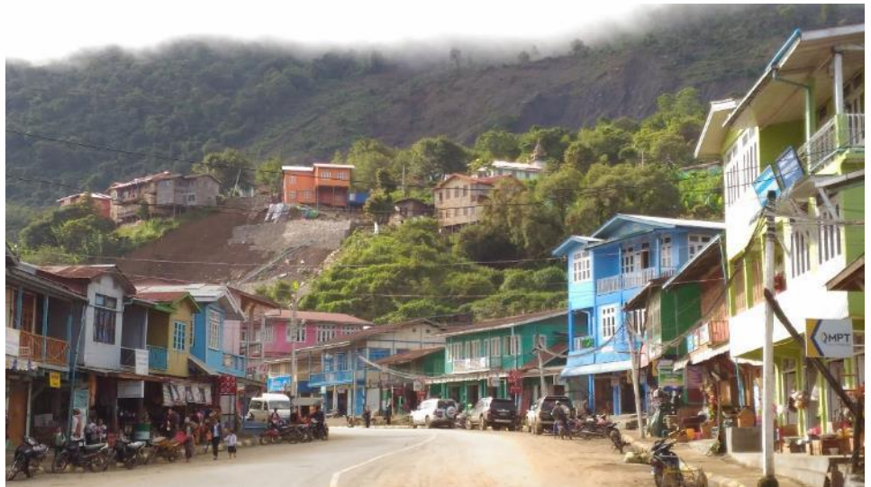
Hakha's colorful wooden houses lie beneath the Rung Mountain, which is an important water source for the residents. (Credit: Carl Middleton)
