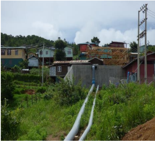
The pipeline and large storage tank that will connect to the Timit Dam, and deliver municipal water to Hakha once commissioned (Credit: Carl Middleton)
